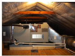
Insulating the roofline (as above, netted cellulose) brings mechanical equipment inside conditioned space
